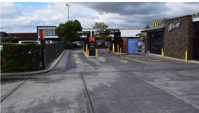
Figure 1: Good natural access control to guide vehicles through a drive-through service zone and use of bollards, colour and signage are further contributors indicating that this area is for vehicles only and not for pedestrian access.
