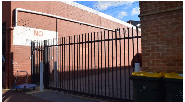
Figure 2: Car park entrance has been target hardened with a spiked steel fence and barbed wire however with adjacent bollards and bins providing readily available scaling points for a motivated offender.
