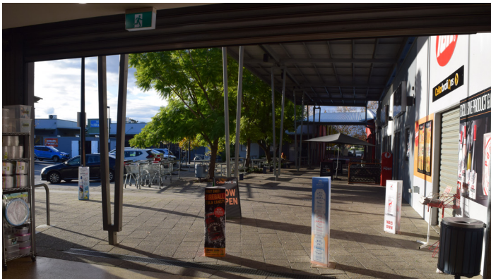
Figure 1: Appropriate use of bollards to restrict or deter vehicle access whilst facilitating pedestrian access and use of signage to cover the bollards creates an alternative dual purpose.
