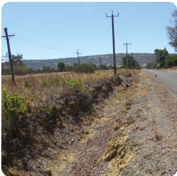
ABOVE: Apple Street Drainage and Power Lines
